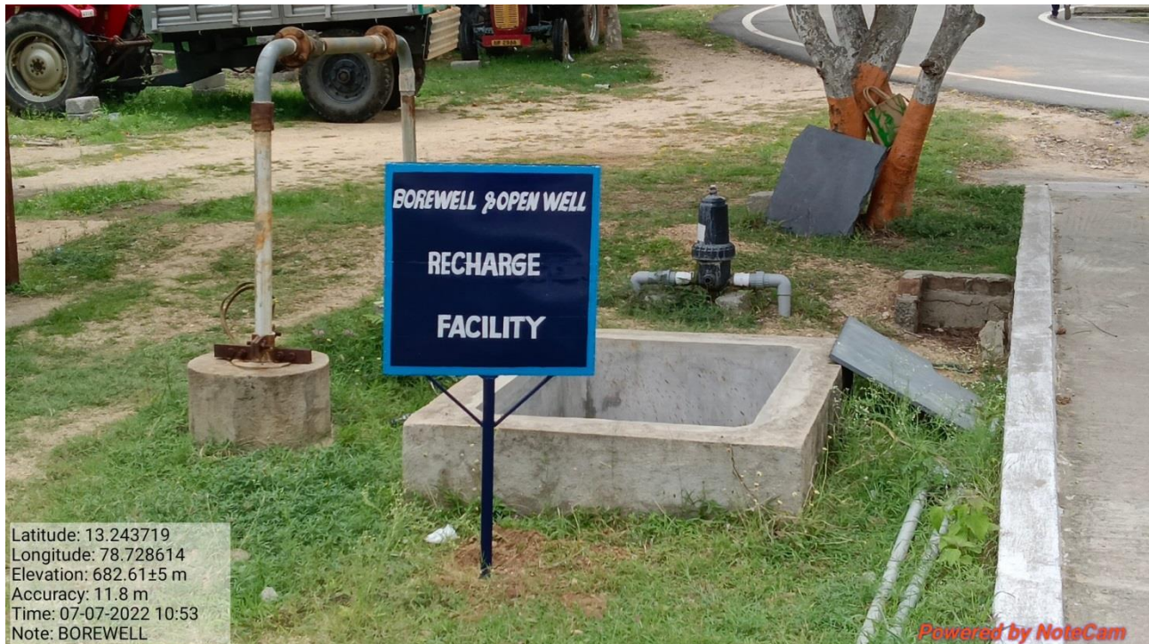
RECHARGE PIT NEAR THE BORE-WELL
